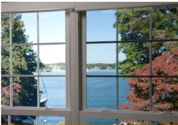
The window on the left has no film; the window on the right does. How much a film alters the appearance of the window (inside and out) depends on a number of variables and is difficult to generalize because there are currently so many different films.
