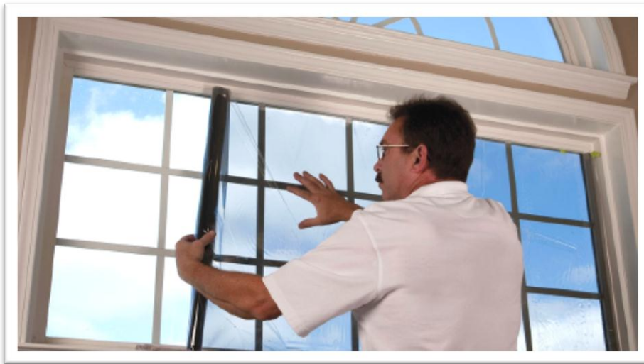
Photo: DOE's Window Retrofit Option Surface-Applied Window Films (Solutia Performance Films)
