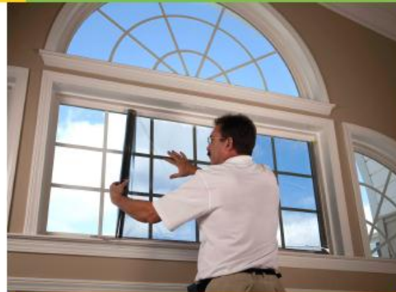
Surface-applied window films can be installed by do-it-yourselfers, but professional installation is recommended. After thorough and specialized cleaning, the installer will apply a solution to the window surface prior to rolling and squeegeeing the film.
