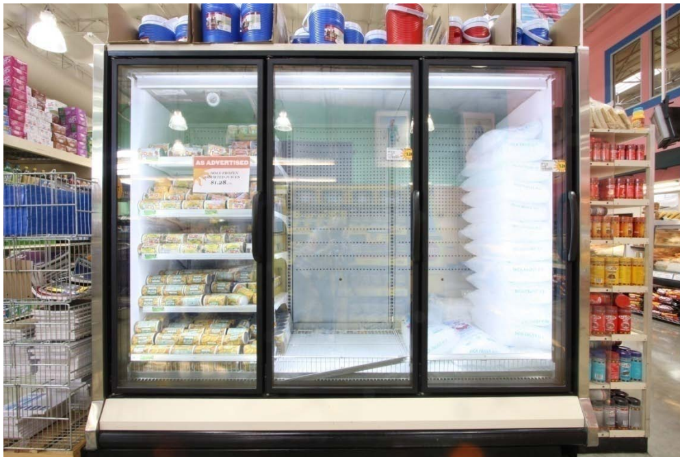
Figure 4-2 LED Lighting (LED Light Bars)
