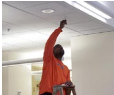
Calibrating a Photosensor
