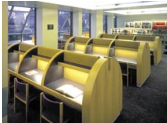
Undershelf task light with local rocker switch in study carrels.
