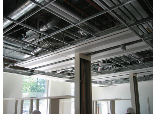
Figure 13. Chilled beams in a T-bar ceiling.
