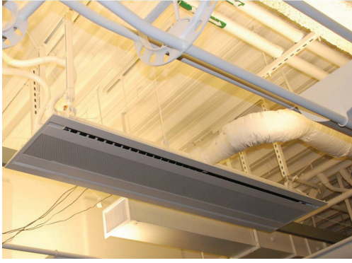
Figure 13. Chilled beams in a T-bar ceiling.
