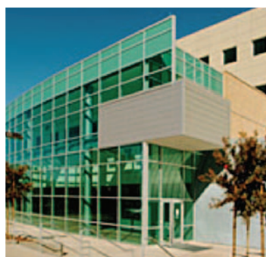
Figure 39. LLNL Terascale Simulation Facility. Photo courtesy of LLNL
