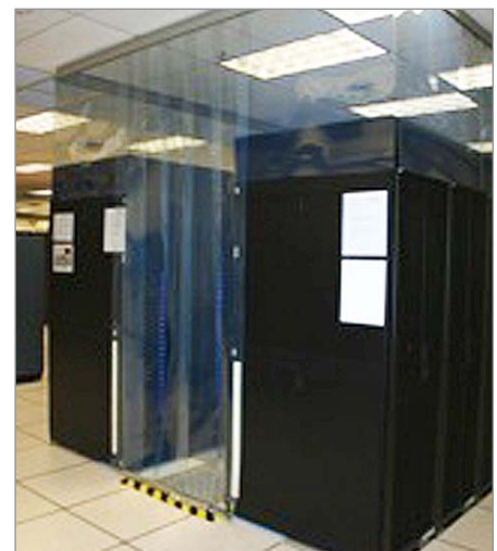
Figure 17. Sandia Labs’ cold aisle containment curtain. Photo courtesy of Sandia National Laboratories
