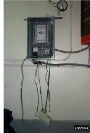
Figure 5.2.3-2: First RE installation
