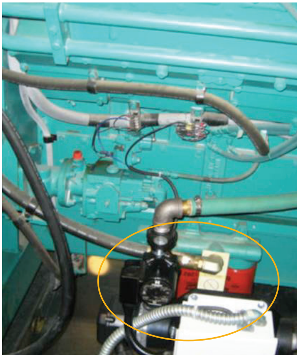
Figure 2: Examples of pump-driven engine block heaters on an indoor and an outdoor standby generator.
