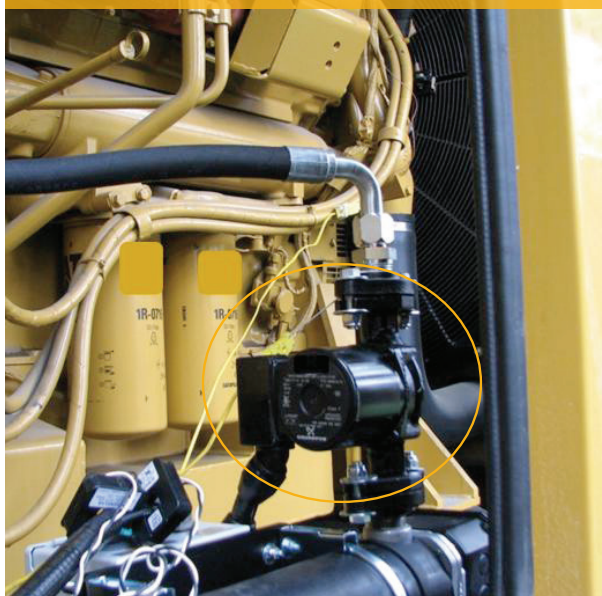
Figure 2: Examples of pump-driven engine block heaters on an indoor and an outdoor standby generator.
